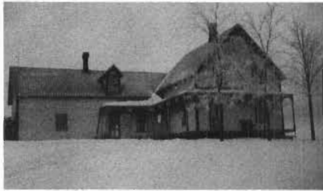
House as it now stands
