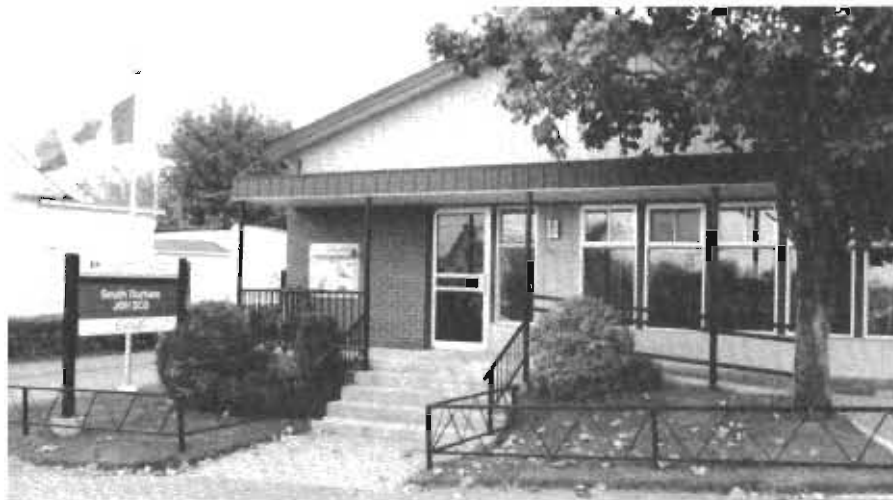
Bureau de poste de South Durham 1988 South Durham Post Office
