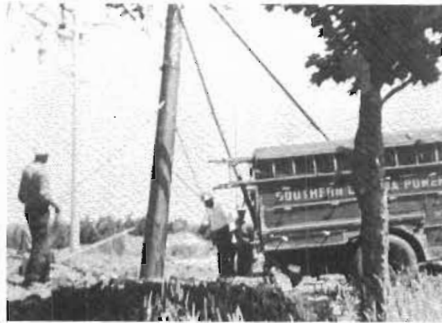
Installation de poteaux circa 1960 Pole installation
