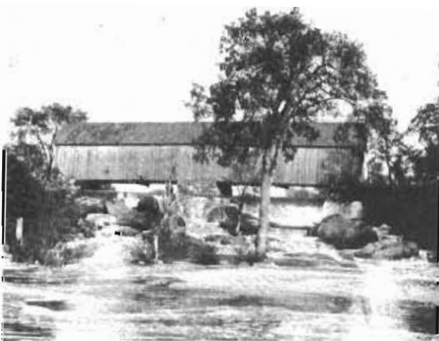
Pont couvert de Lisgar (1860-1945) Lisgar covered bridge
