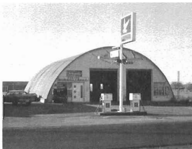
Station de service (1980)
