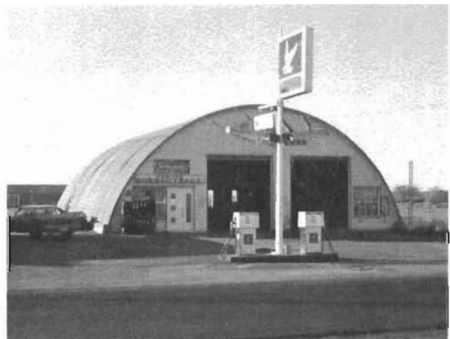
Station de service (1980)
