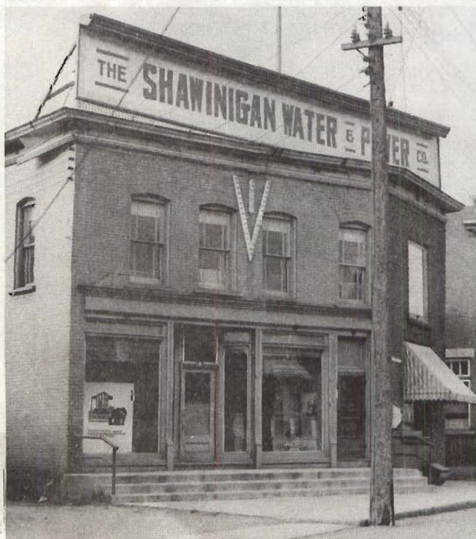
1940-1950 - Shawinigan Water and Power, rue Notre-Dame
