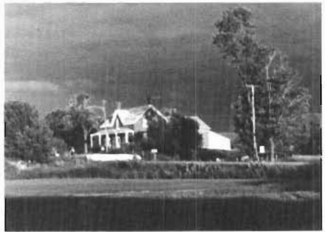
Maison typique d'Ormstown Typical Ormstown home
