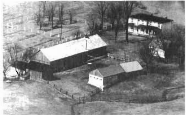
An aerial view of the house which was destroyed by fire
