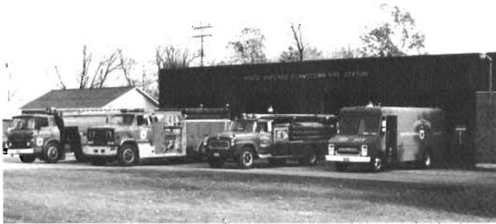
La caserne / Fire Station built in 1976
