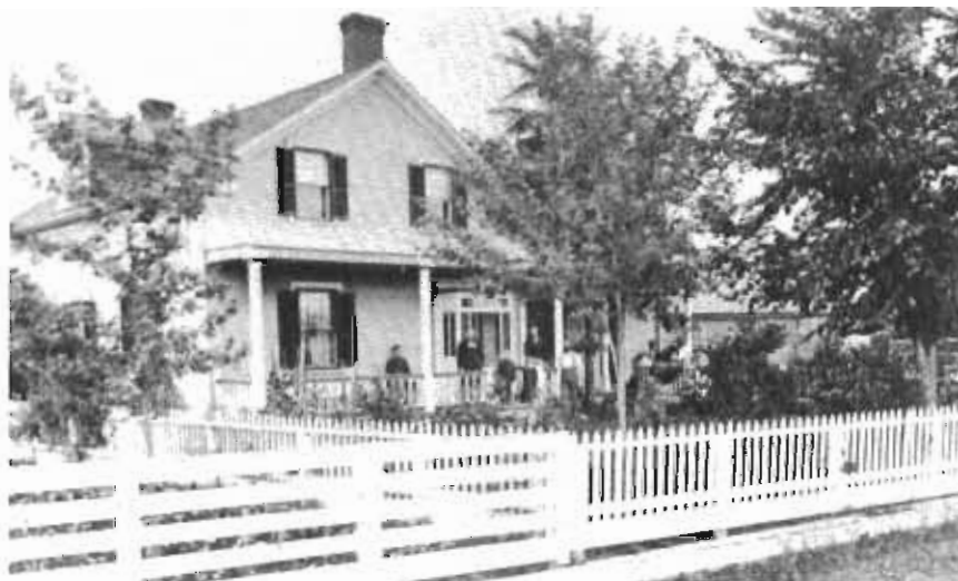
The Homestead house, 72. Lambton St.
