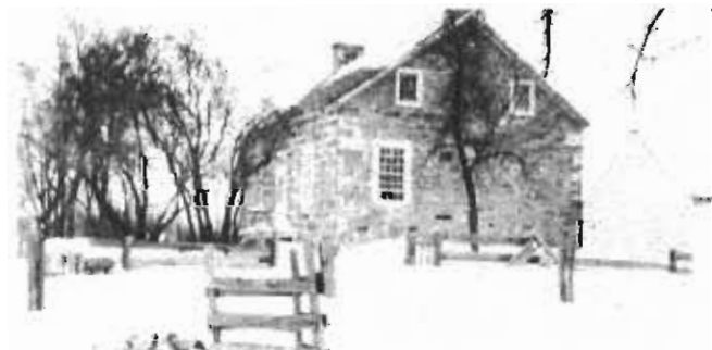
picture of house - 1919, before roof was raised
