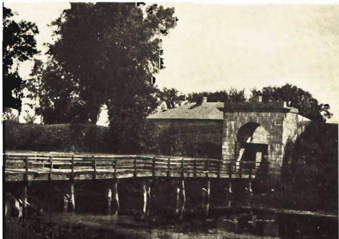
MAIN ENTRANCE, NORTH SIDE
