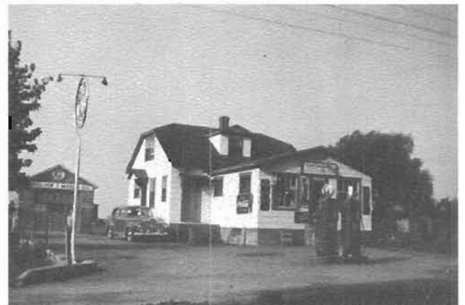
Restaurant-garage, au village de Saint-Blaise
