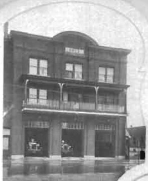
STATION DE POMPE - FIRE STATION
