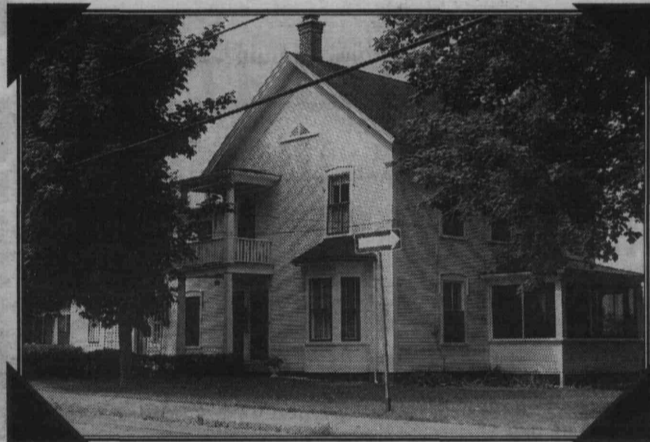
William Stevenson Residence 114, rue William
