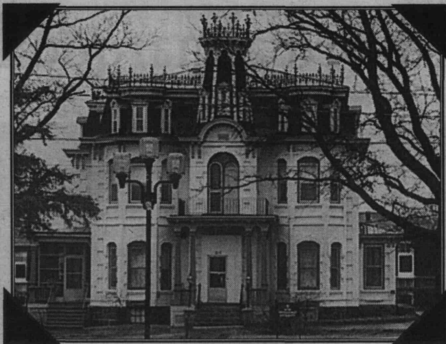
G.K. Nesbitt Residence 215, rue Sud
