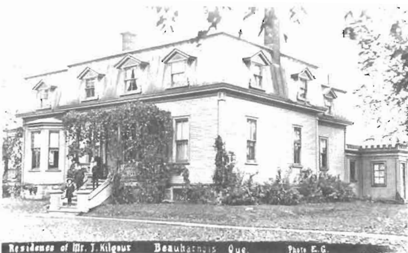
Residence of Mr. J. Kilgour Beauharnois Que. Photo E. G.
