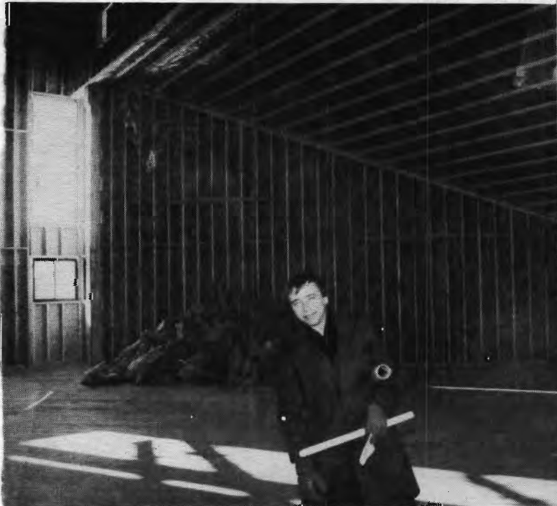
Fr. Brad McGovern with building plan on hand with smile of hope that the building will be finished on time.
