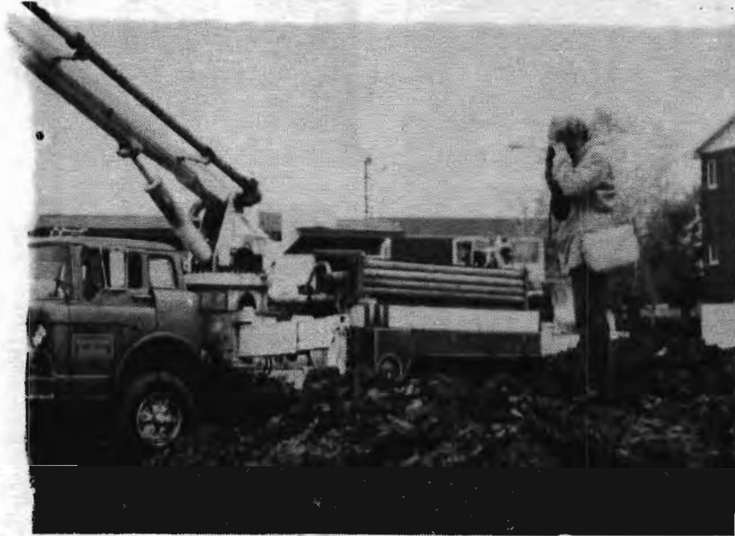
GERTHIE RAHN capturing the excavation
