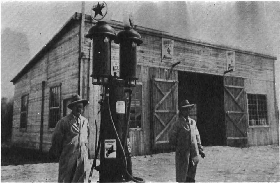
Station Service Pion et Poulin (1948)
