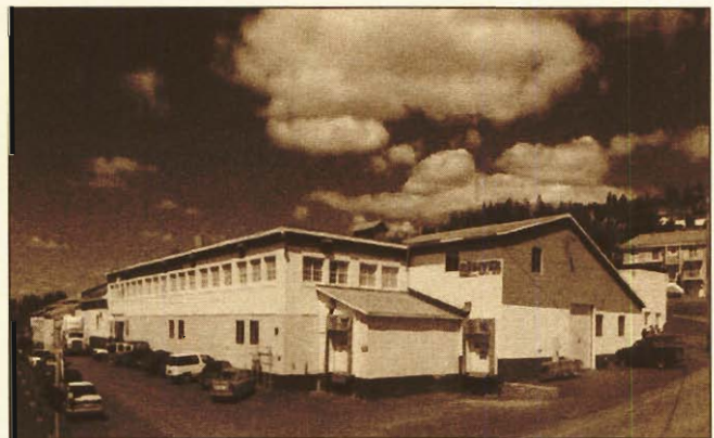
Usine B (112 route Fraser)
