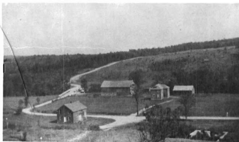
Lower left: Thomas Davidson's house. Upper middle: Harvey Bullard's house. Lower right: Foundation to grist mill. Millfield area.
