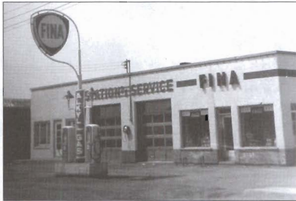
Garage Station de service , Victorin Vaillant, 1955
