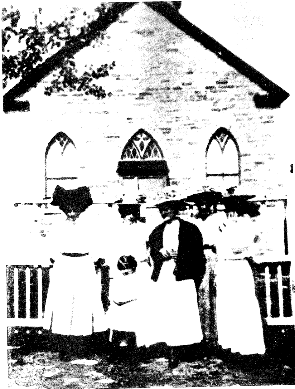
St Andrew's Presbyterian Church by the end of last century.
