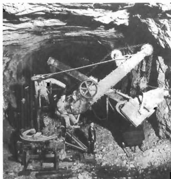
What in those days were modern powered shovels were used to assist in the mammoth excavation job for the tunnel.
