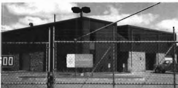
Station de pompage
