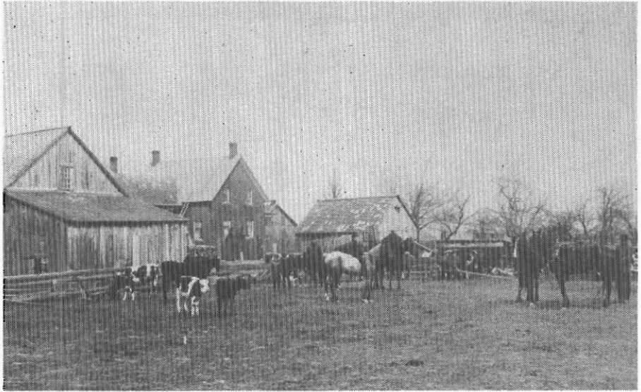
Reid homestead -- Franklin's Corners
