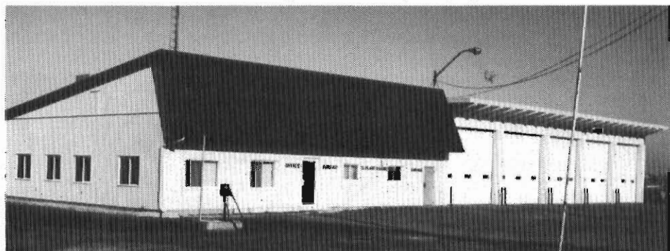
South Plantagenet municipal offices (left), municipal garage (right)
