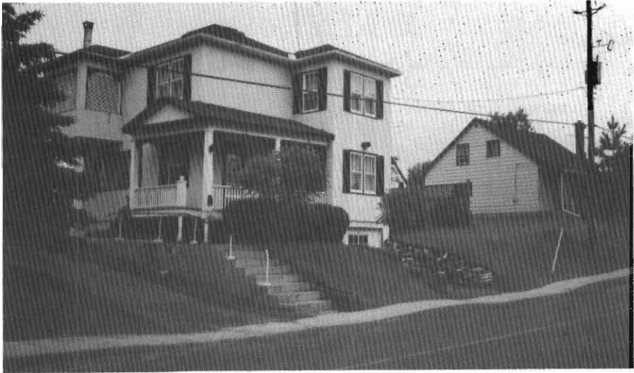
This house was built by Célisier Campeau in 1950. Albert Bourgon bought it in 1972 and sold it in 1987.
