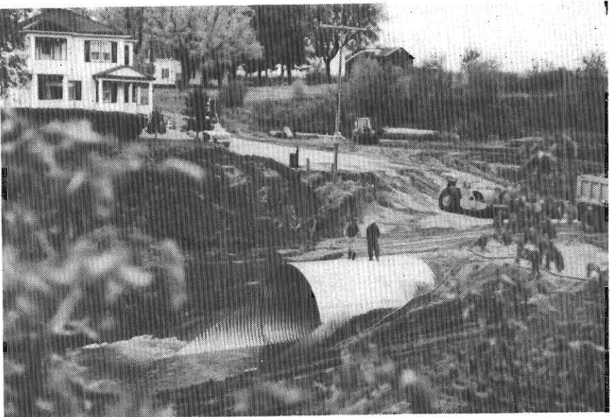
Detour ahead -- bridge under construction - 1984 Dean Ryan, James McCullough
