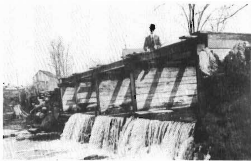
A close-up of the the dam at Morrison's Mill.
