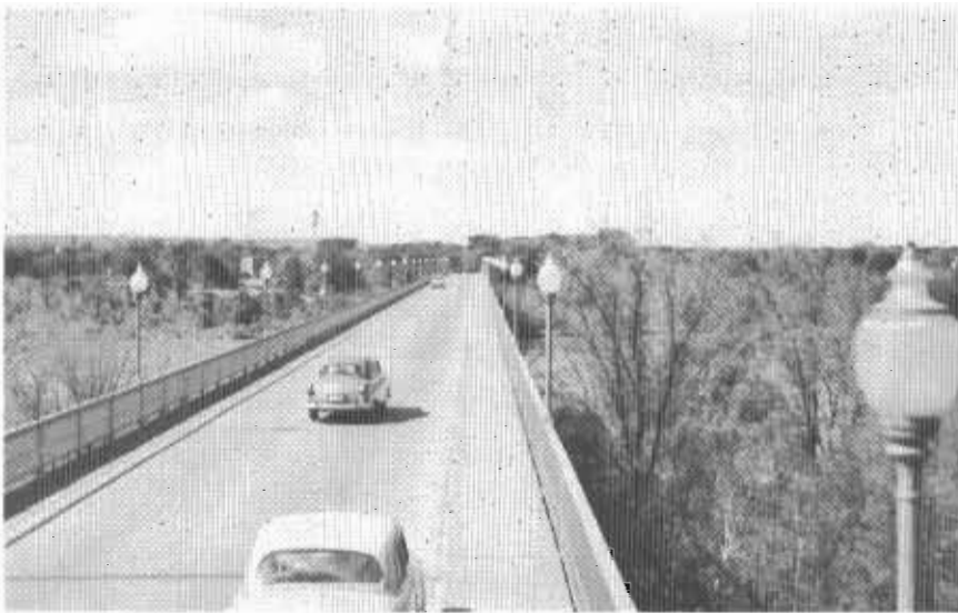
Views of the Perley interprovincial bridge before modification
