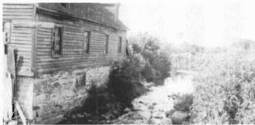
Morrison's Woollen Mill, long after it had been boarded up. The outline of "raceway", bricked over, can be seen at the lower left of the foundation, parallel to the creek.
