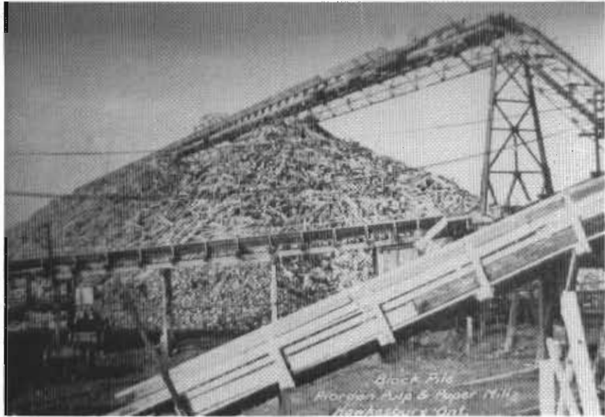
A typical "block pile" at the Hawkesbury Mill.
