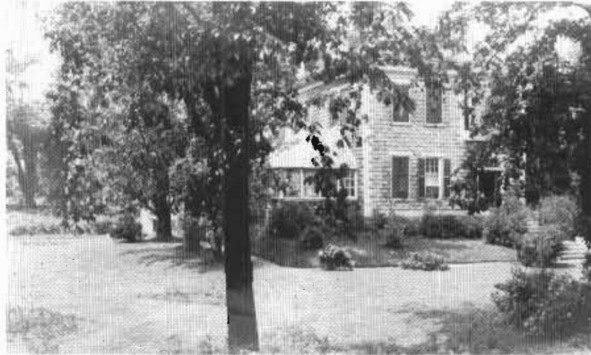
The Thomas Ross house, later part of the (old) Hawkesbury General Hospital.
