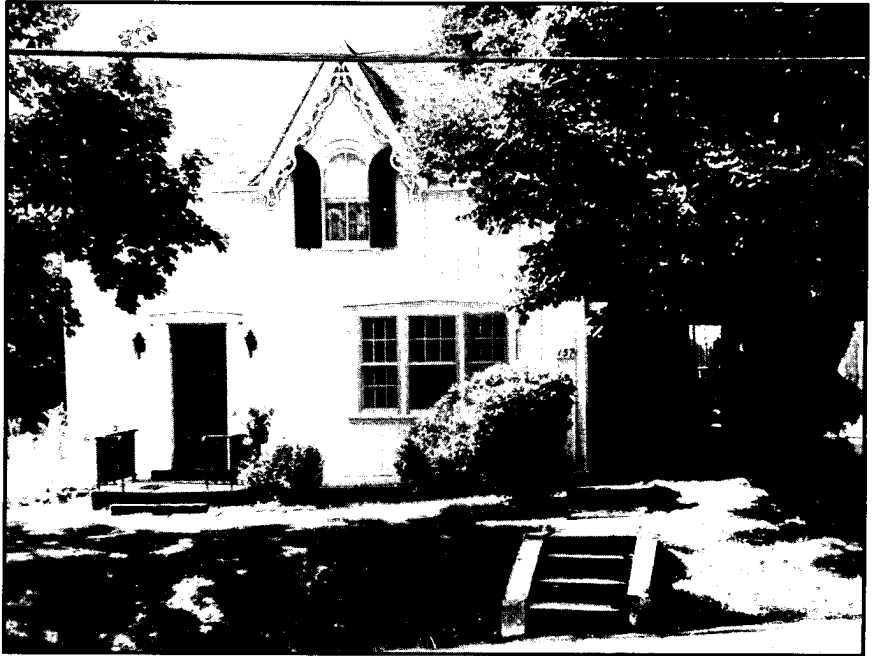
Kirby House, 357 Dundas Street, Summer 1977
