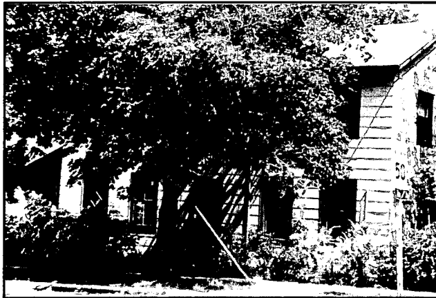
Double House, Summer 1977. Covered with modern siding, the house was last rented to the Lewis and Downs families before demolition c.1982.
