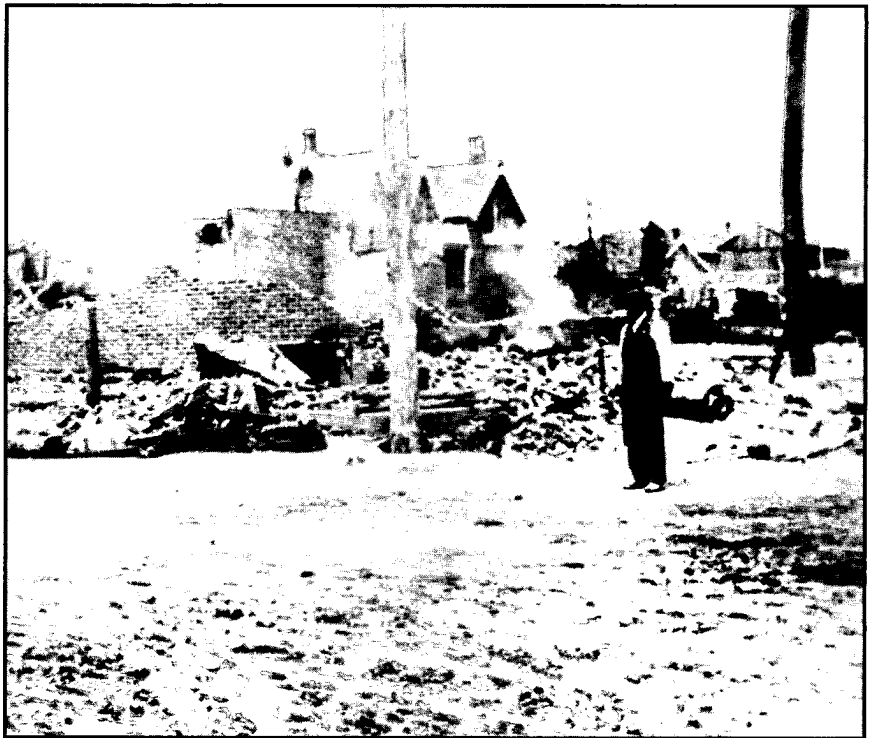
Fire damage on Dundas Street looking north-east to Chestnut Grove, May 25, 1915.
