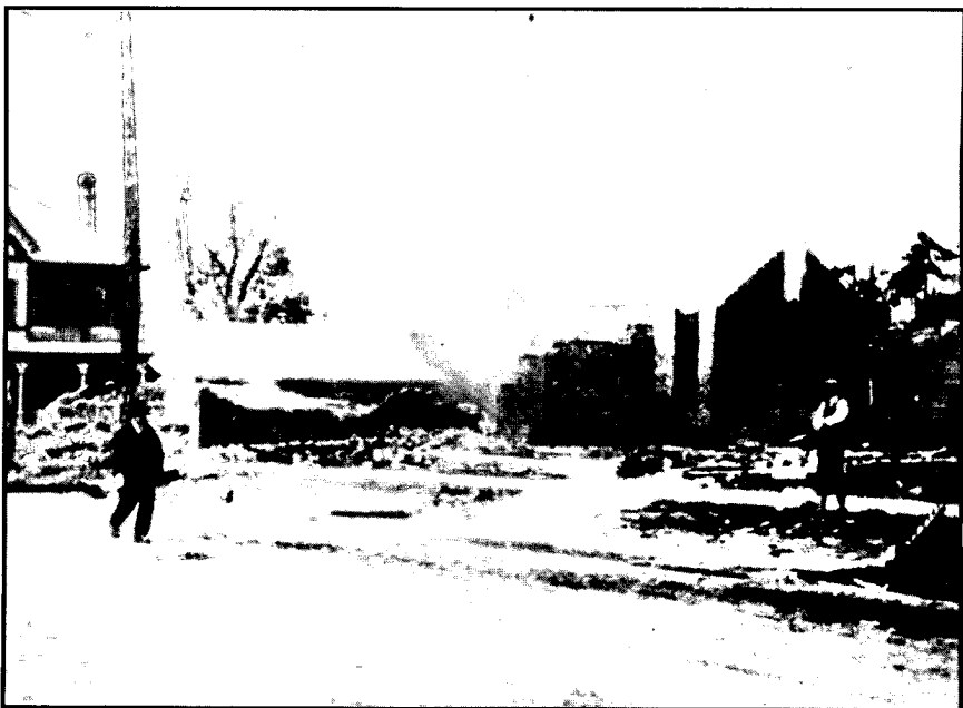
Fire damage on Dundas Street looking west, May 25, 1915.
