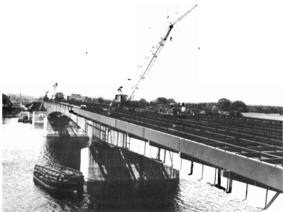
Works on one of the bridge's span in 1963. (Coll. N.C.C.)
