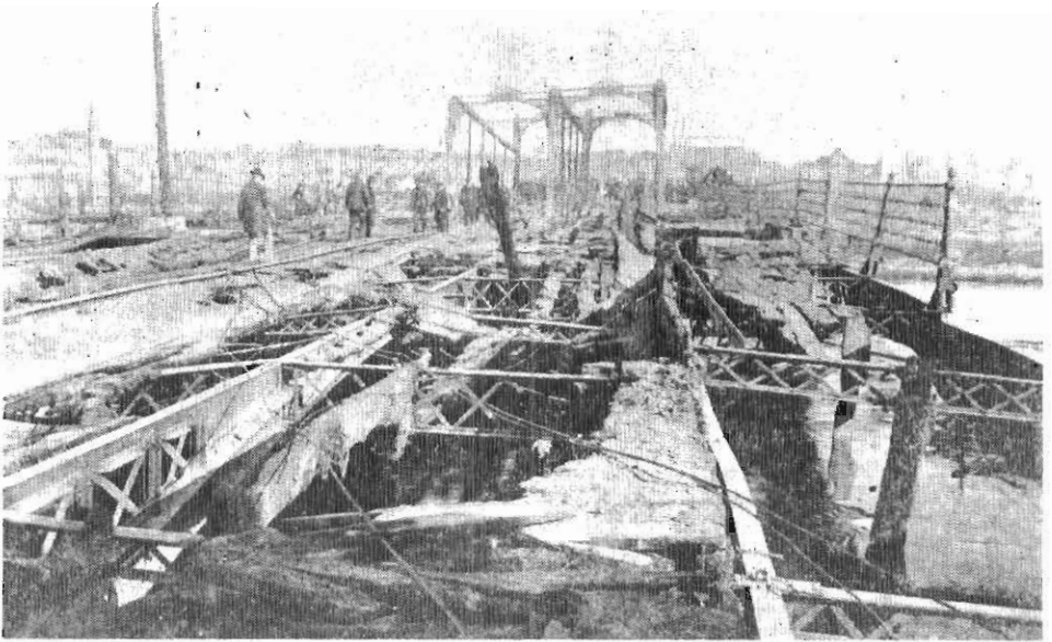
The bridge's destruction from another point of view. (Coll. Ottawa City Archives)
