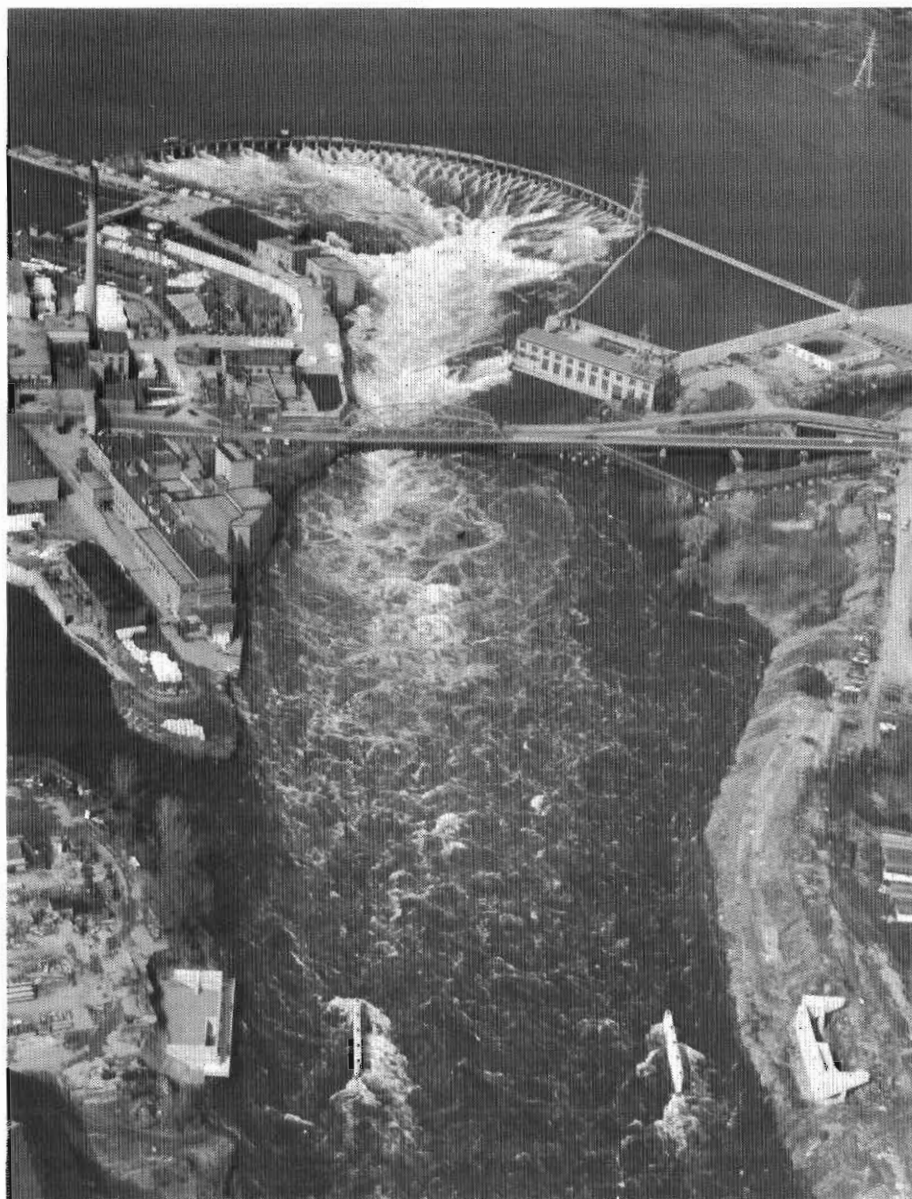
In the foreground, pillars of the Portage bridge in march 1972. (Coll. Ottawa City Archives)
