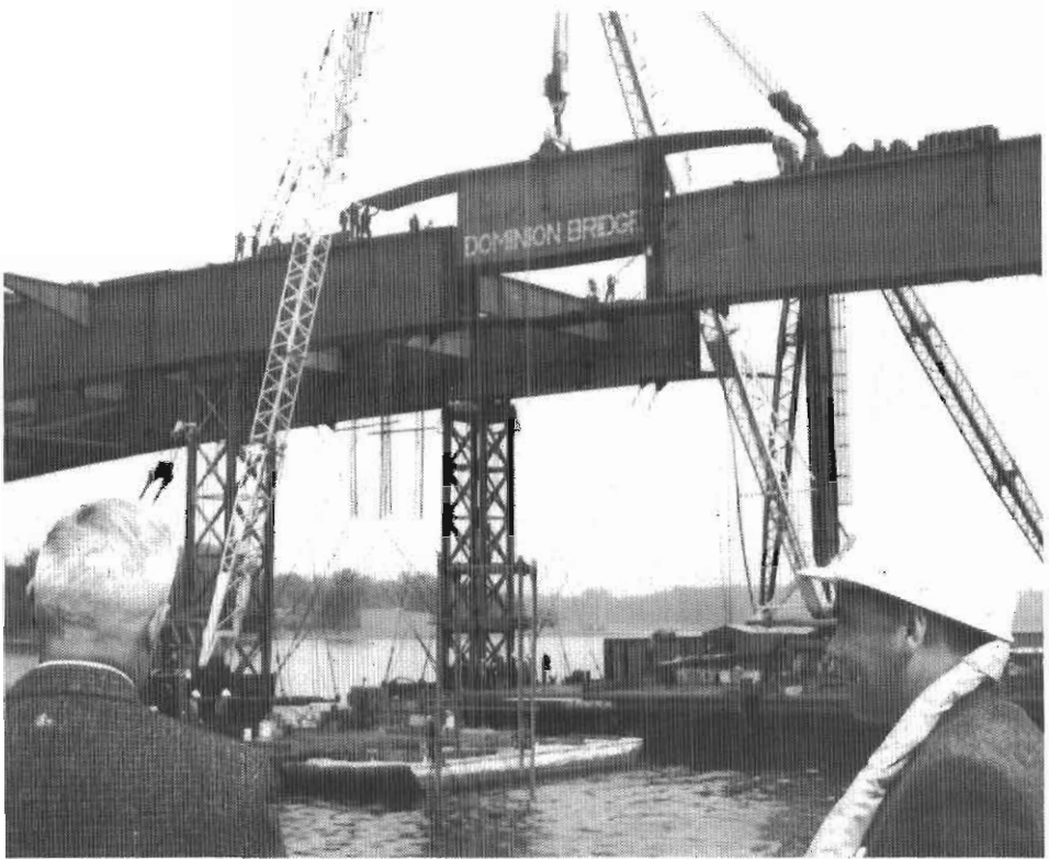
Installing the main span in Spring 1964. (Coll. N.C.C.)
