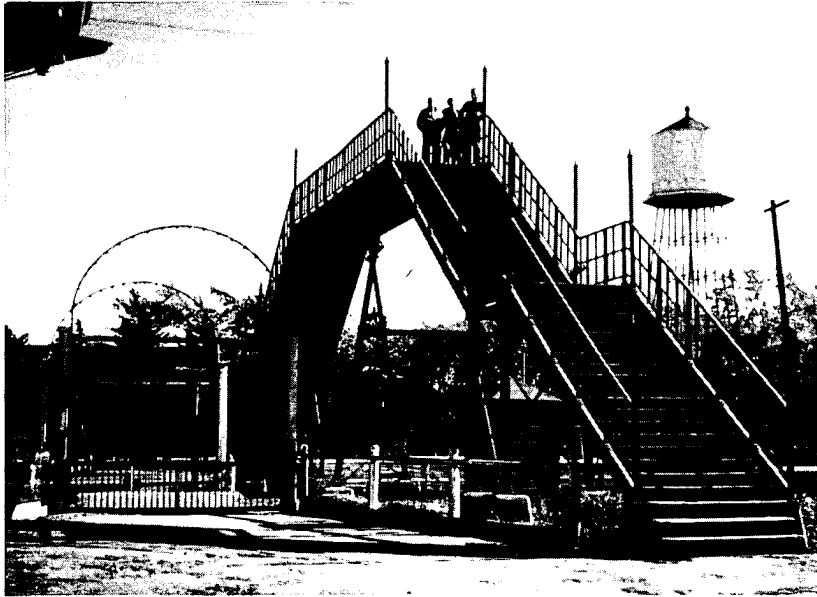
The bridge over the C.P.R. tracks, the gates and water tank in Britannia Park, 1952.
