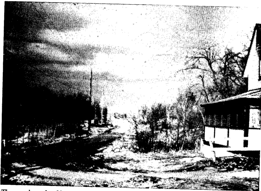
The road to the filtration plant under construction, 1959. The cottage on the right, the Ranch, was built in 1895 and owned by J.R. Smith.
