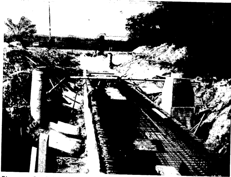
Pinecrest Creek being put underground near the river, August 1966.
