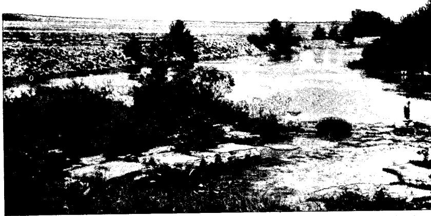
The lower section of the canal showing the old crib work to the left. (1950)
