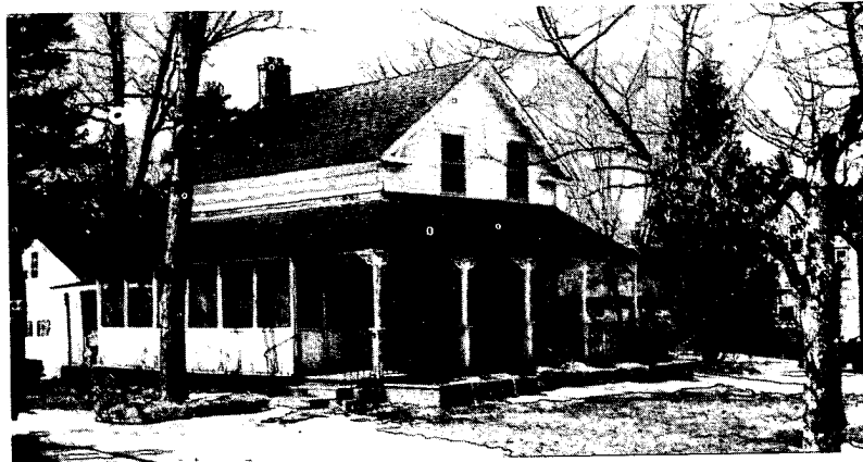
80 Bradford Street, once the manager's house for the mills at the Deschênes Rapids. Later it became part of "The Grove".
