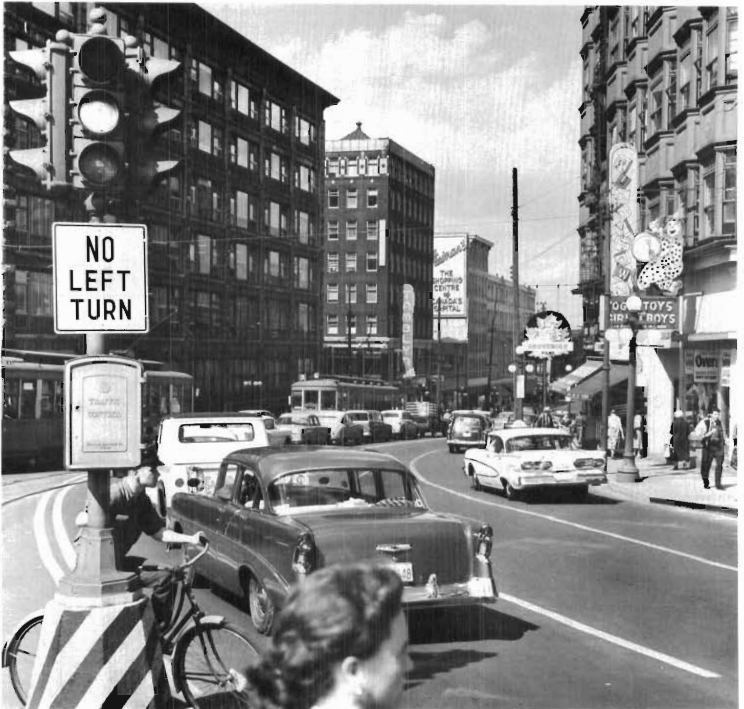
RIDEAU STREET, LOOKING EAST, c. 1958
