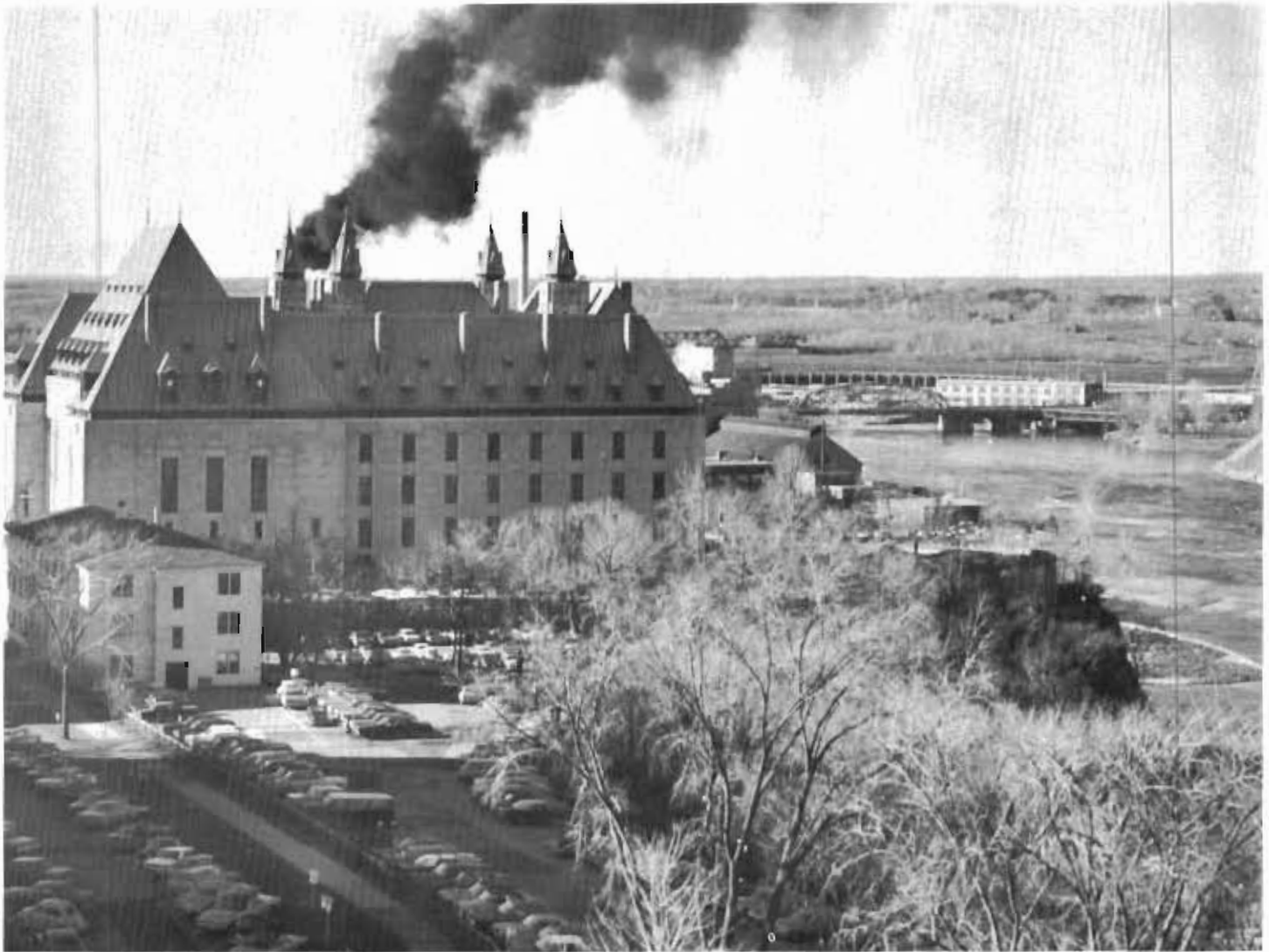
THE OTTAWA RIVER AND THE SUPREME COURT BUILDING FROM THE WEST BLOCK, 1970
