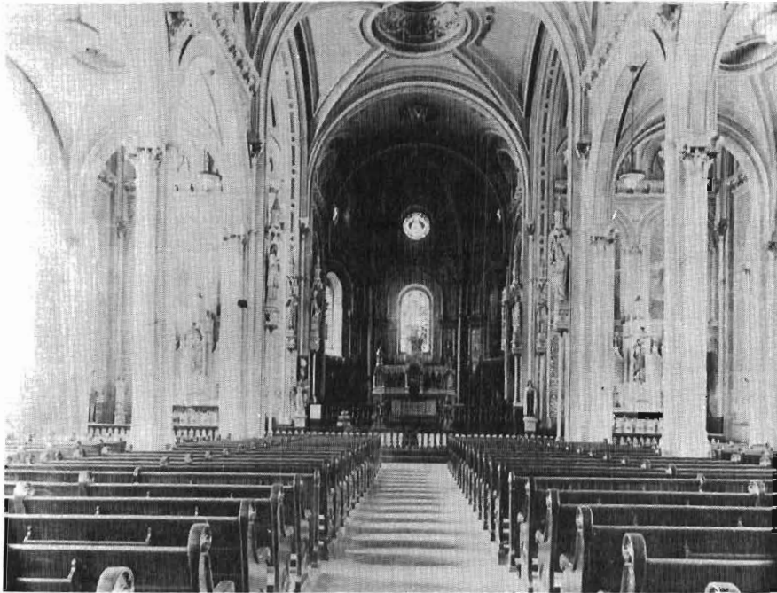
ST. COLUMBAN'S INTERIOR PRIOR TO THE EARTHQUAKE
