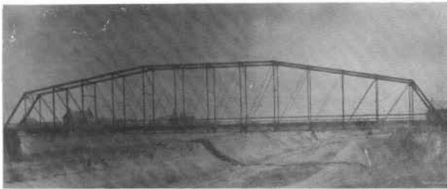
The bridge across the new canal from Victoria St., and the partial digging of the canal.
