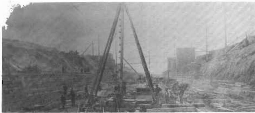
The building of the canal. Note the bridge abutments, new canal.
