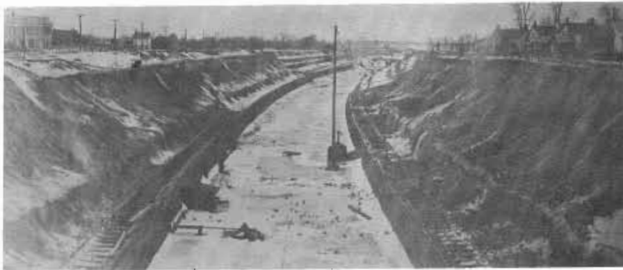
The building of the new canal in the early days. Note the earthen banks and the installation of the first part of the crib work.
