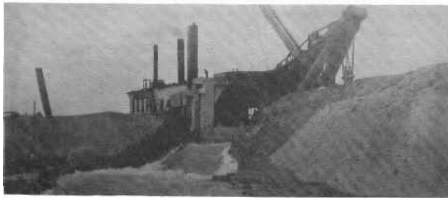
The water coming into the new canal.
