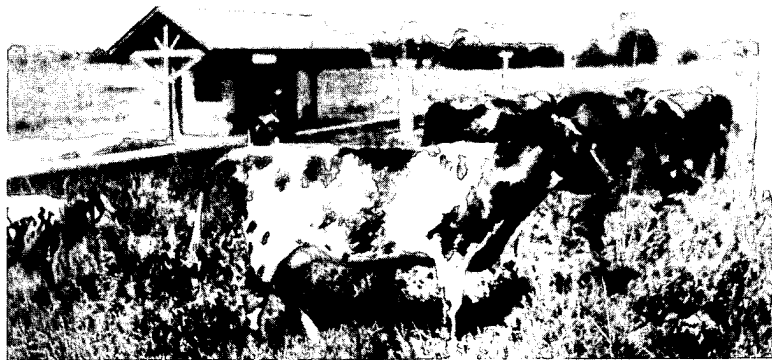
ABOVE: Original G.T.R. milk loading station, Wicklow, c. 1860. Photo loaned by W. Finley
