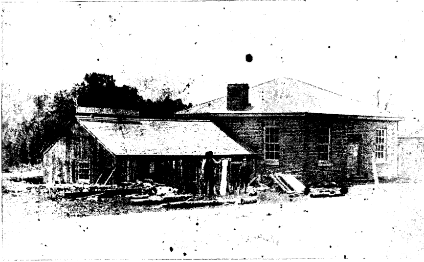
Taylor Pump Works, Shelter Valley, c. 1900. Photo loaned by Carolyn Taylor.
