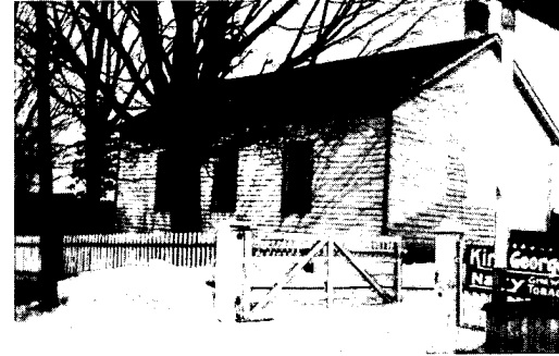
ABOVE: Centreton school. Photo loaned by Margaret Ryerson.
