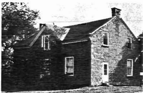
Stone house built by Thomas Ellis on Dalkeith Street.
