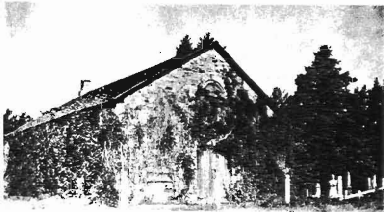
After the first Presbyterian Church in Pakenham was burned in the 1840's, this building of local sandstone was erected through the efforts of Mr. Mann and his congregation. Courtesy J. T. H. (Bud) Gordon, Manotick.
