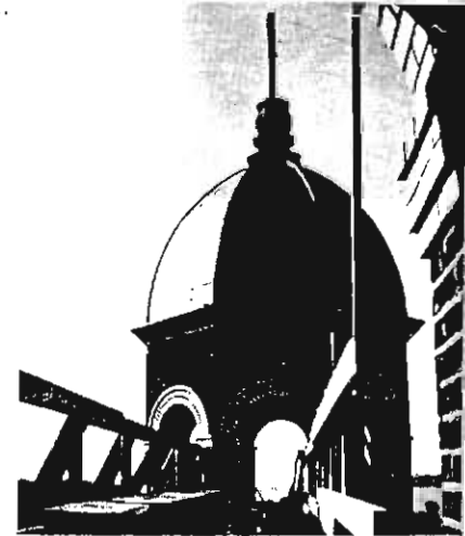
View of Church Tower during renovation, 1984
