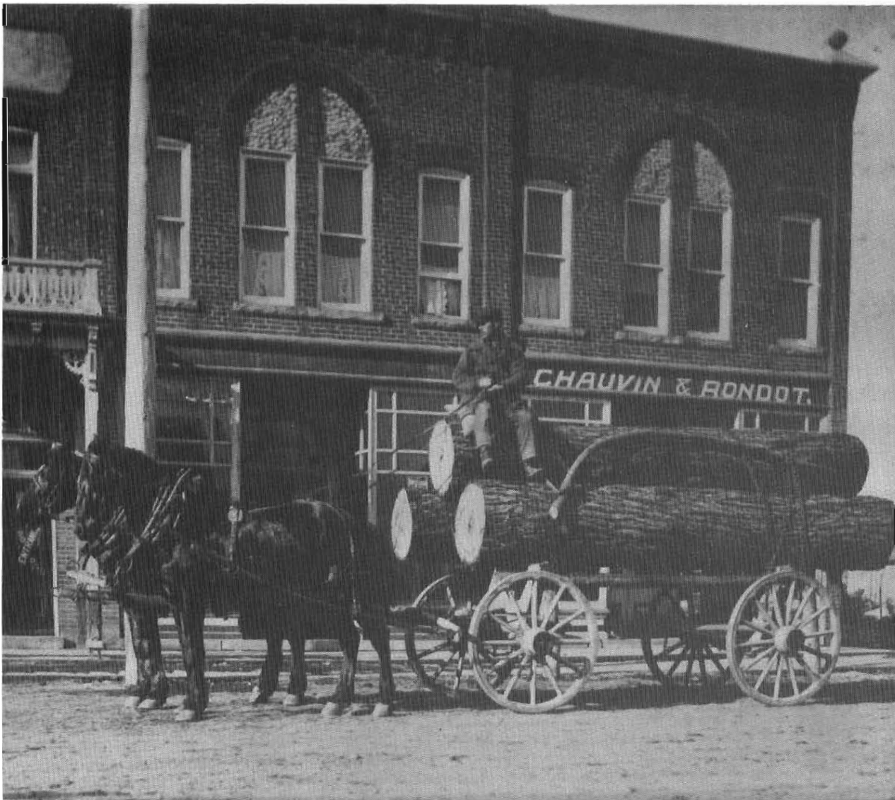
In 1897 Calixte Renaud drove one of 85 teams hauling logs to the Ainslie Mill in Comber. These were made into barrels and other related products.
