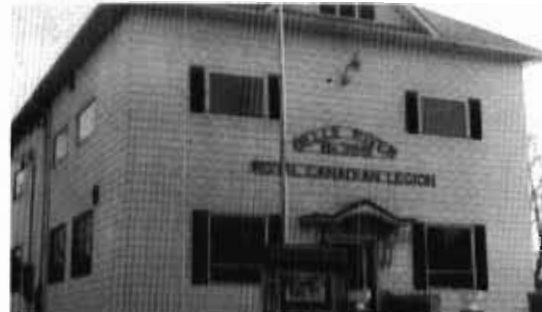
St. James High School was purchased by the Royal Canadian Legion in the spring of 1960, and extensively renovated to become one of the finest Legion facilities in Essex County
