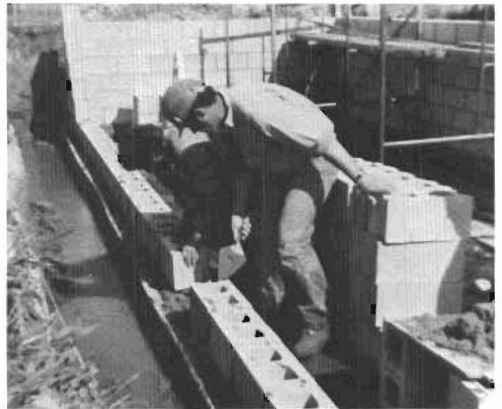
Construction TNT Frères Timony
