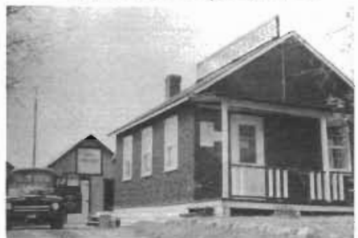
The Deputy Chief Forest Ranger Headquarters, built c.1930, was located in the area of today's access road. This base was in service until about 1955 when a new Lands and Forests Headquarters was constructed. George Boyle was a Deputy Chief Ranger here in the early years. Quartier général du chef-adjoint des gardes forestiers, construit c.1930 dans les environs du chemin d'accès actuel. Le bureau a servi jusque vers 1955, quand on a construit un nouveau quartier général des Terres et Forêts. Les premières années, George Boyle était chef-adjoint des gardes forestiers.
