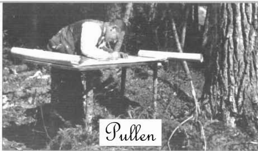
July 1906: E.F. Pullen. Construction of the National Transcontinental Railway. (National Archives) / E.F. Pullen. Construction du Chemin de fer National transcontinental. (Archives nationales)
