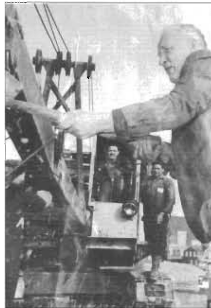
c. 1950: Sod turning for the construction of the arena and Legion hall. Front: Tom Moore Sr. Rear: Ira Evans, crane operator Al Davidson, Fern Gervais.
