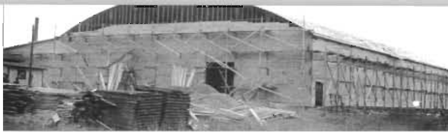
c. 1951: Construction of the arena./Construction de l'aréna
