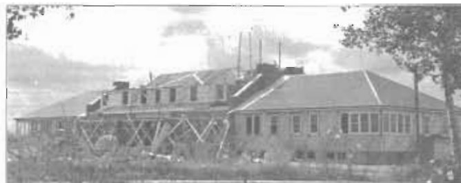
Sept. 9, 1949: Construction of the 4 th hospital Construction du 4 e hôpital
