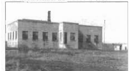
The cookery (see boiler house on right)
