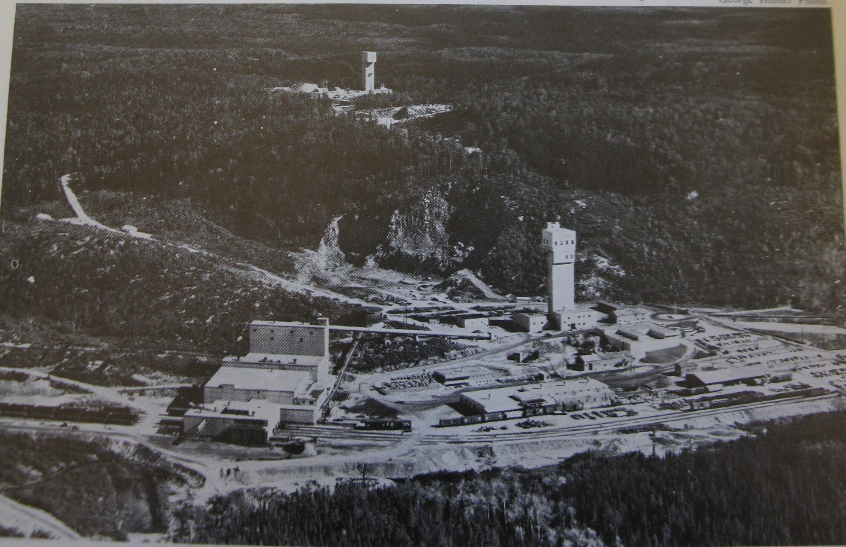
Shown in this aerial picture are the principal surface installations of Noranda's Geco Mine. The two headframes, both equipped with friction-drive hoists tower high over the other buildings and the surrounding bushland. George Hunter Photo.
