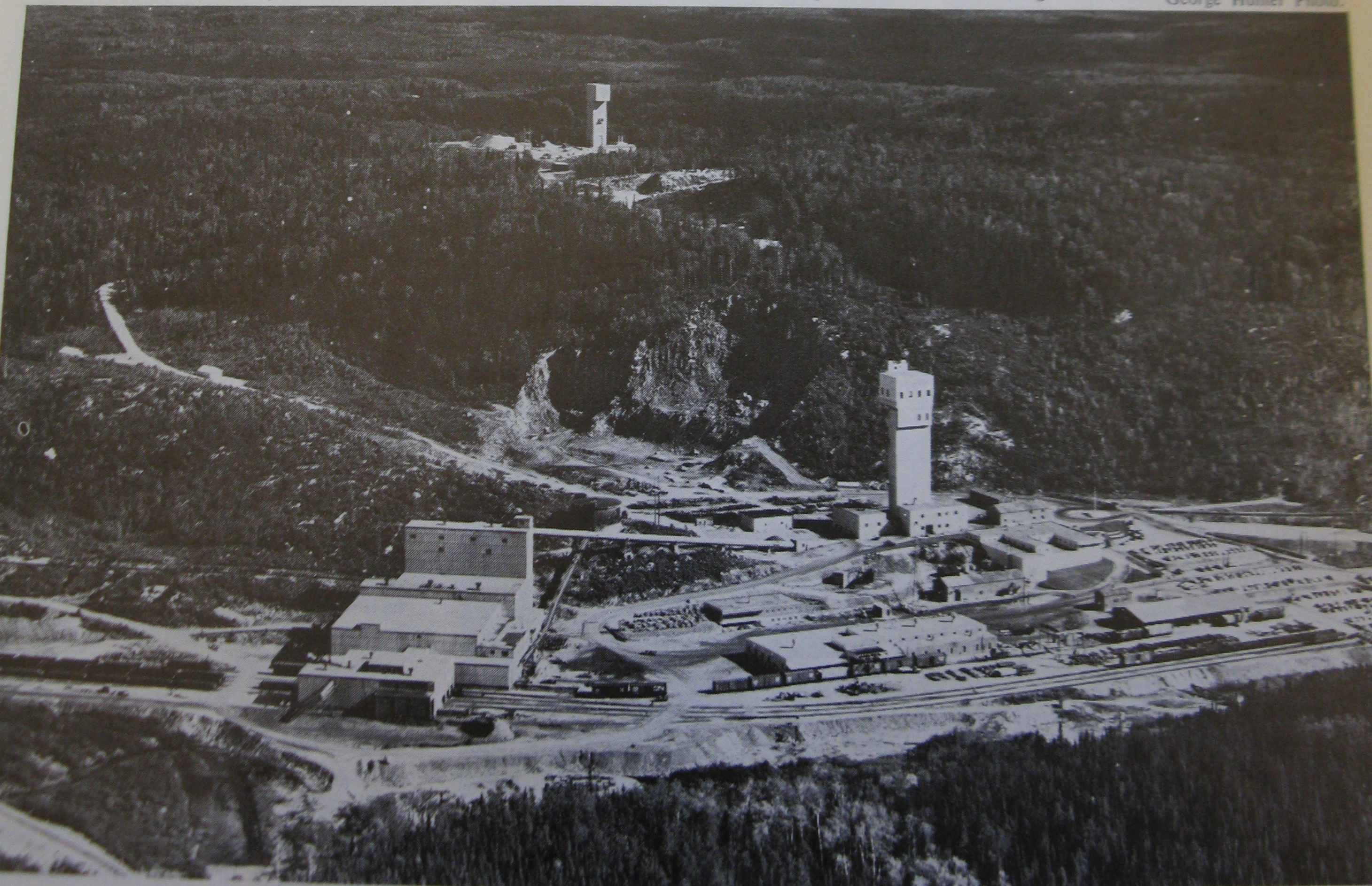
Shown in this aerial picture are the principal surface installations of Noranda's Geco Mine. The two headframes, both equipped with friction-drive hoists tower high over the other buildings and the surrounding bushland. George Hunter Photo.
