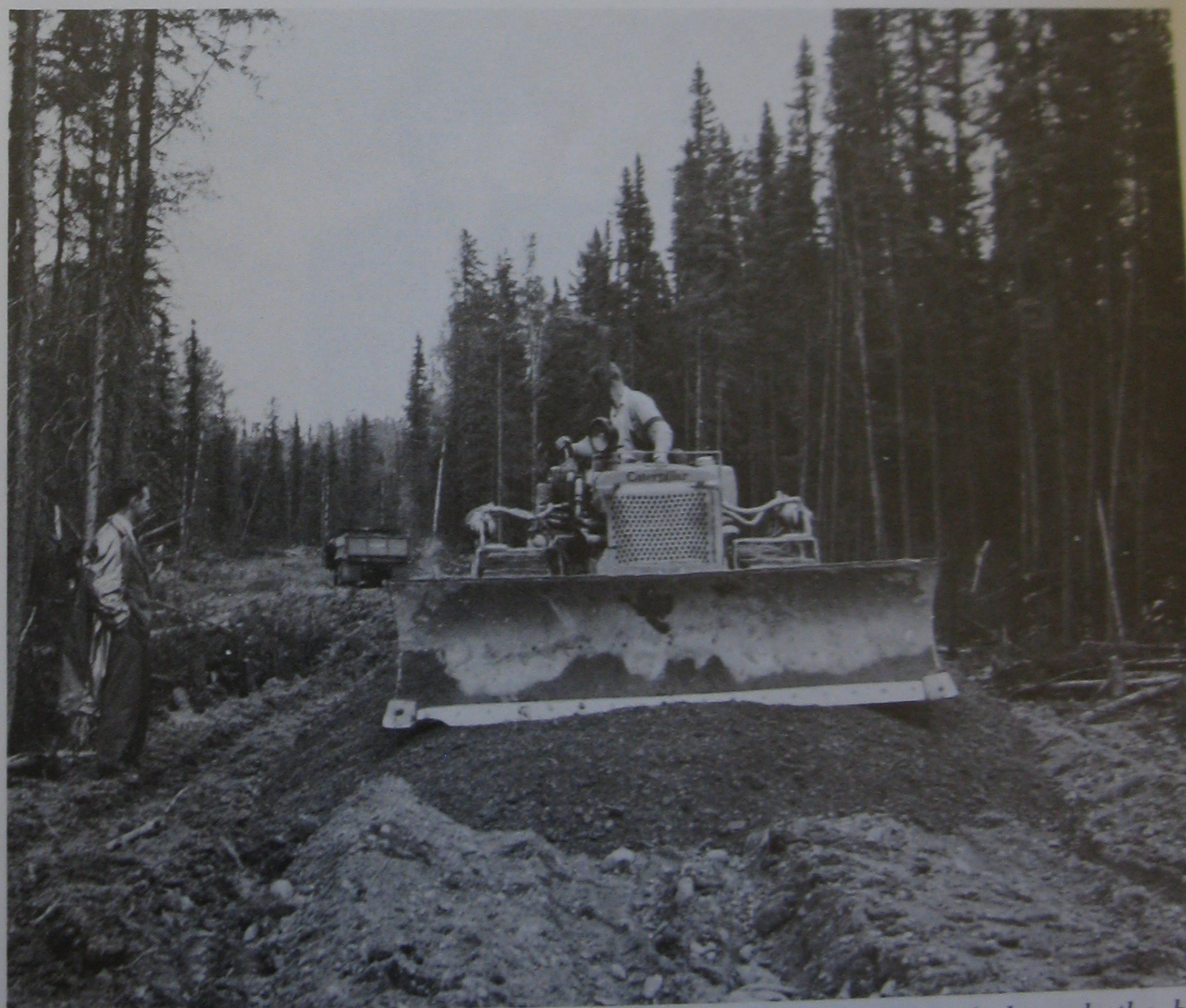
The access road into Manitouwadge from the south was bulldozed through the bush in quick time after the decision was taken to establish mining operations.
