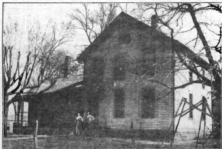
HOMESTEAD OF ADAM FRITZ (THIRD BUILDING), PILOT TOWNSHIP SECTION 17.
