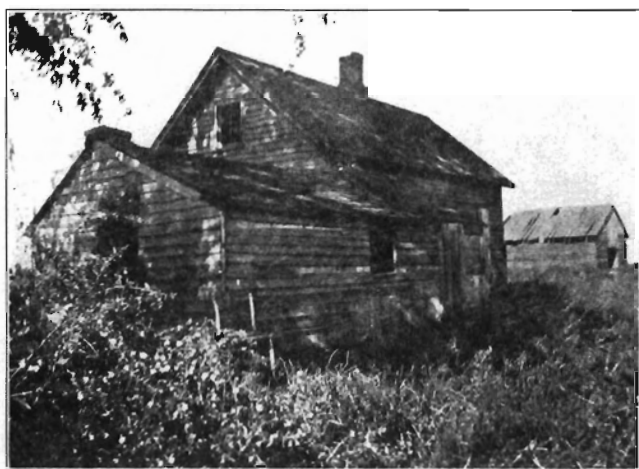
HOMESTEAD OF GEORGE O'NEIL PILOT TOWNSHIP, SEC. 36.
