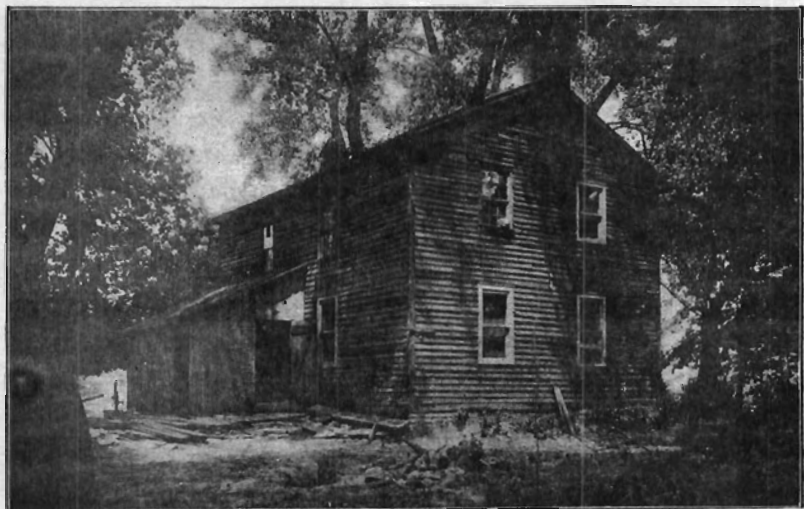
BUILDING ERECTED IN 1850. AT PRESENT (1920) SAME CLAP-BOARDS, AND FOR THE MAJOR PART SAME WINDOWS AND SHINGLES. SALINA TOWNSHIP SECTION 28. HERTZ'S GROVE.
