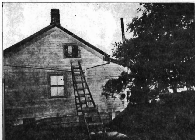
DWELLING HOUSE OF MATTHIAS TREMBLAY, TOWNSHIP OTTO, SECTION 29.
