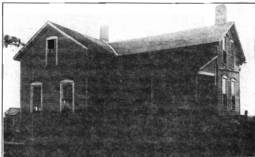
HOMESTEAD OF FRANCIS STUDER (1845)...PILOT TOWNSHIP SECTION 16.
