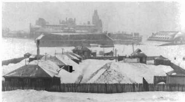
Overall view of one of the loading and assembly workshops on the Plains of Abraham (Cove Fields) January 1899 Photo. Public Archives of Canada
