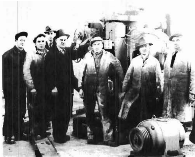
Moving equipment from the workshops on Côte du Palais circa 1964 Photo: Parks Canada collection
