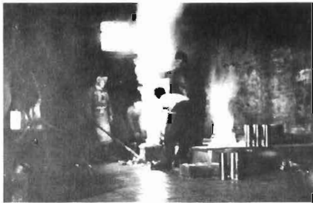
Workers preparing to do a casting Circa 1910 Photo: Parks Canada collection
