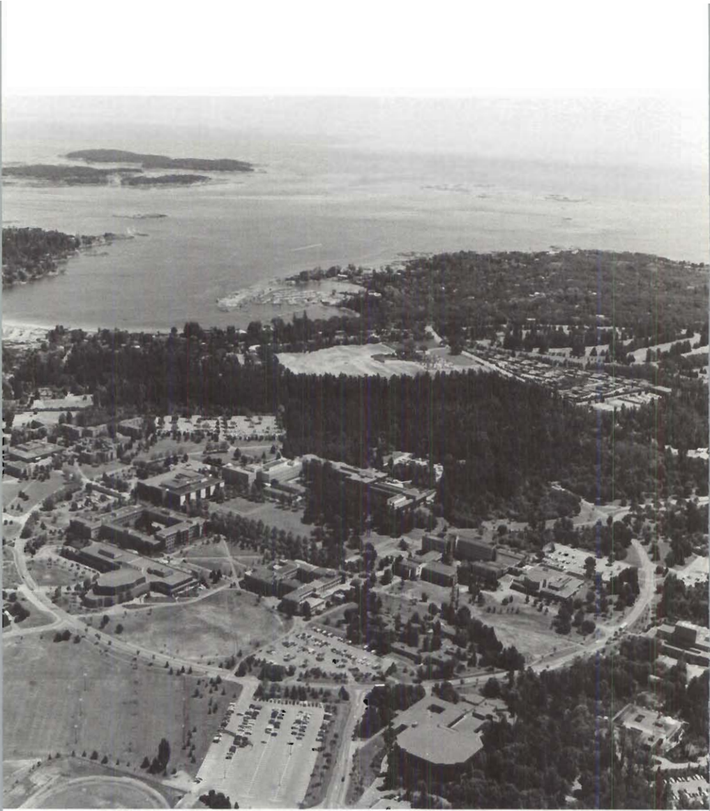
Aerial View of the University of Victoria. #0207870411 Photo by: Don Pierce, UVic Photo Services.
