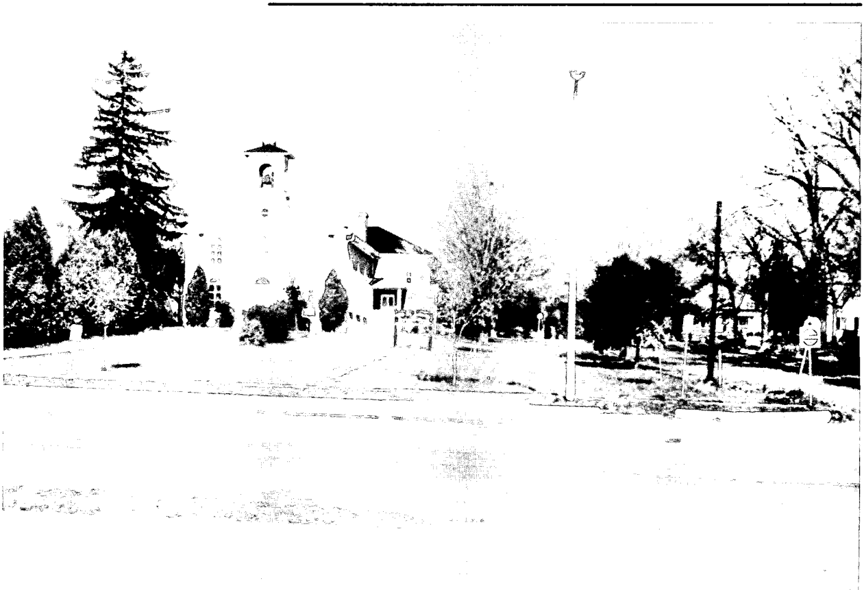
Fig. 4.6 Colborne Presbyterian Church plaza today (built 1830).
